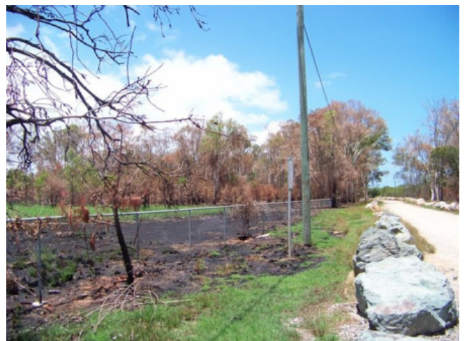
Fire ravaged area showing signs of recovery after the rain - Photo R Smith
